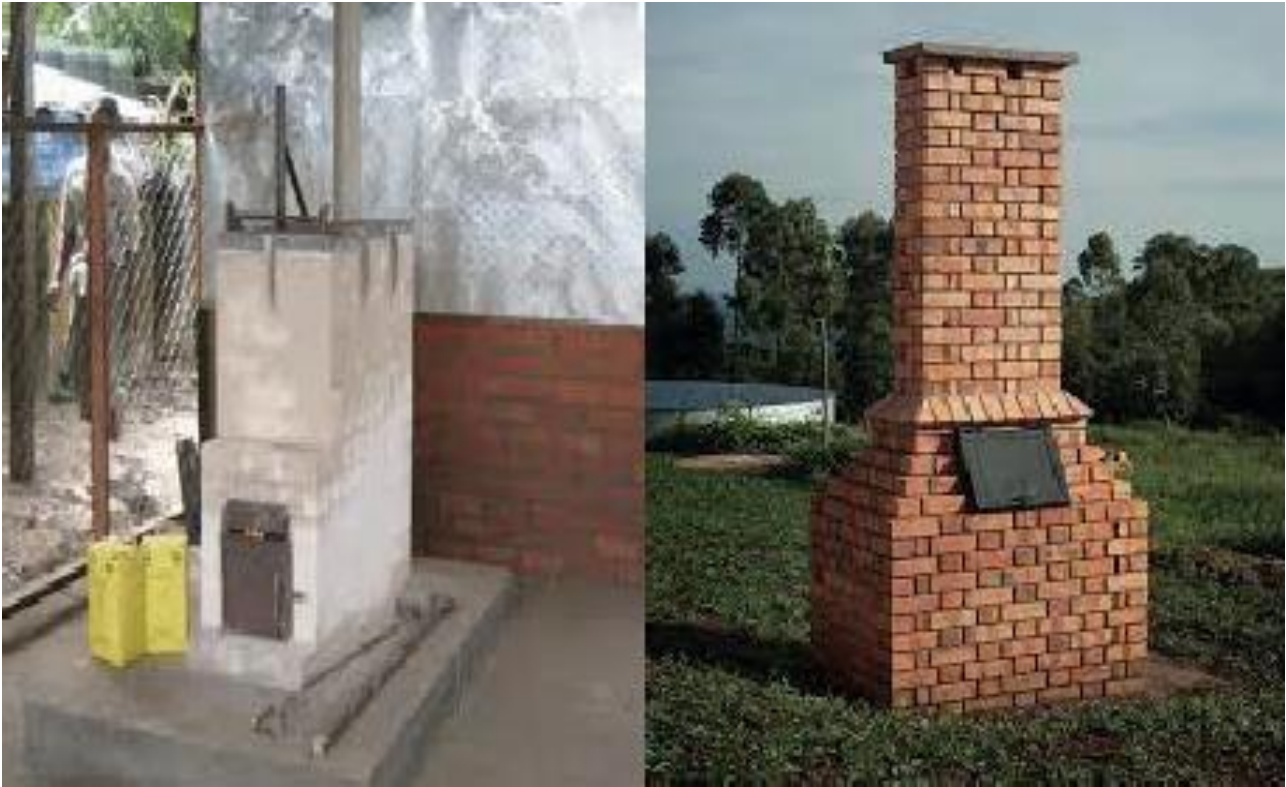
Fig 5.3. Incinerator with fence and ash pit.
