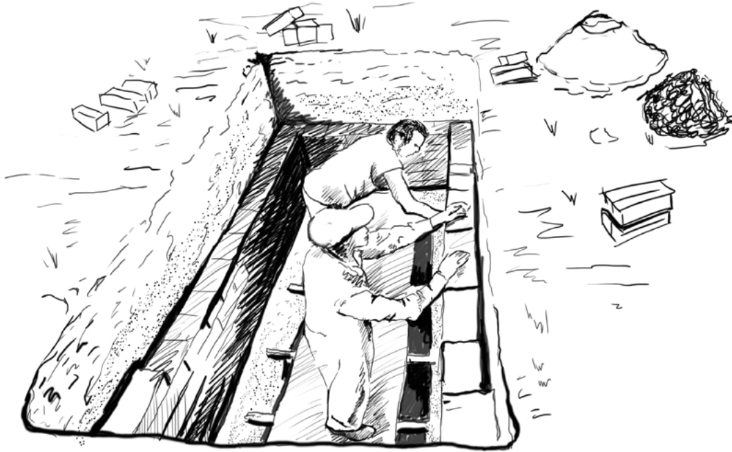
Figure 13: Pit lining with bricks
