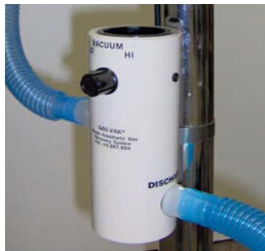
Figure 4.36: Open scavenging system
